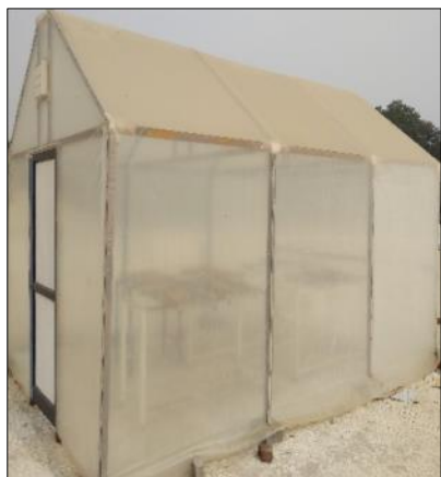
Fig 2: Side view of greenhouse dryer
