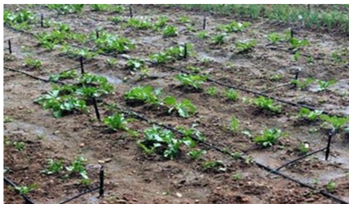
Fig 3.1: Laying of laterals in Papaya plot
